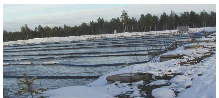
Municipal plant in Poland, 4,200 PE 60
