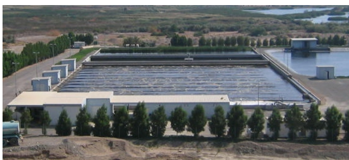
Municipal plant in Saudi Arabia, 100,000 PE 60
