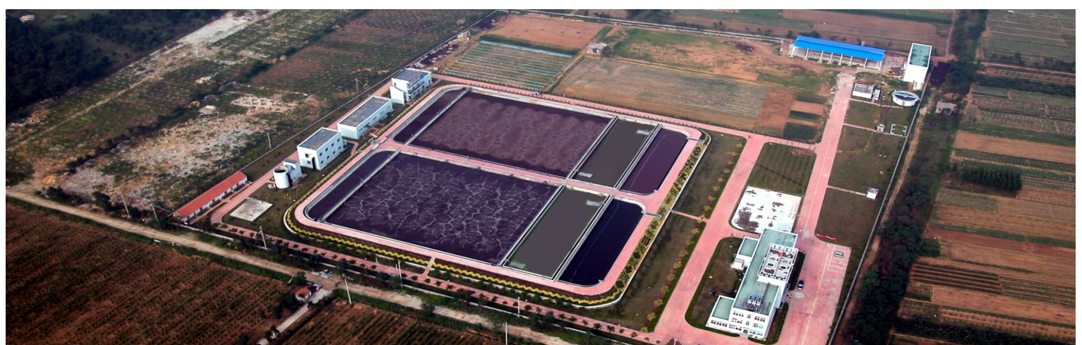
Municipal plant, 40,000 m 3 /d - 200,000 PE 60
